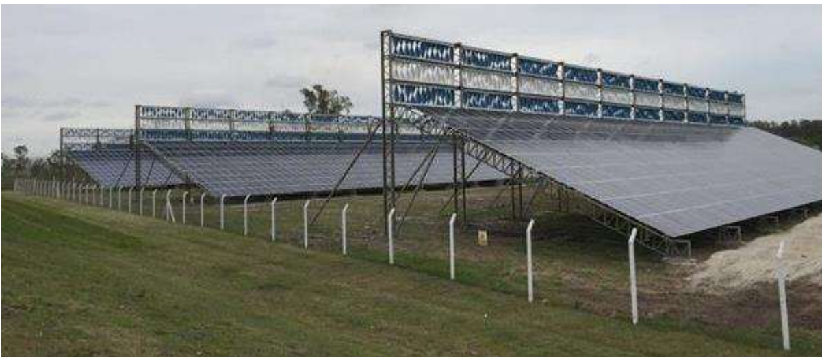
40Kw Power Mil installation for Mini Grid application.
