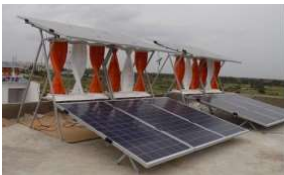
A 10 KW Hybrid Installation @ Industrial area Shamherpet, Hyderabad
