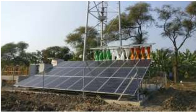
11Kw Installation for Telecom Tower
